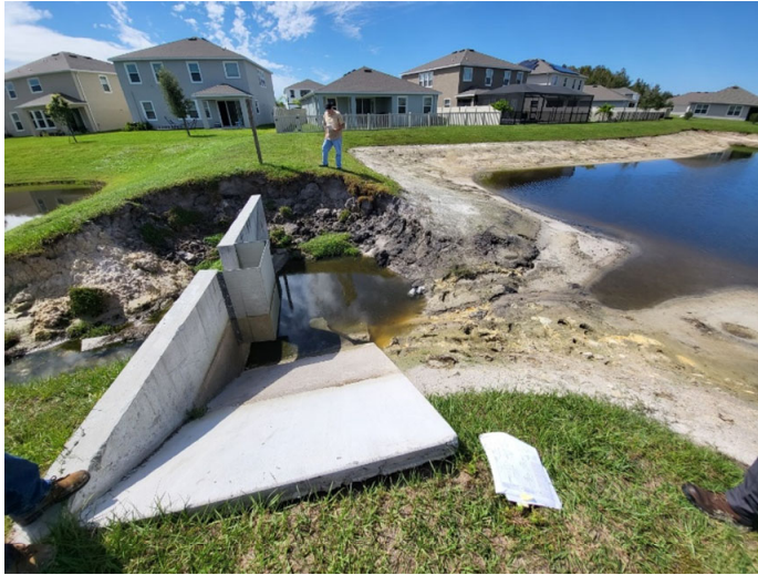
Photo showing cracks on north side of concrete structure just below the weir.
