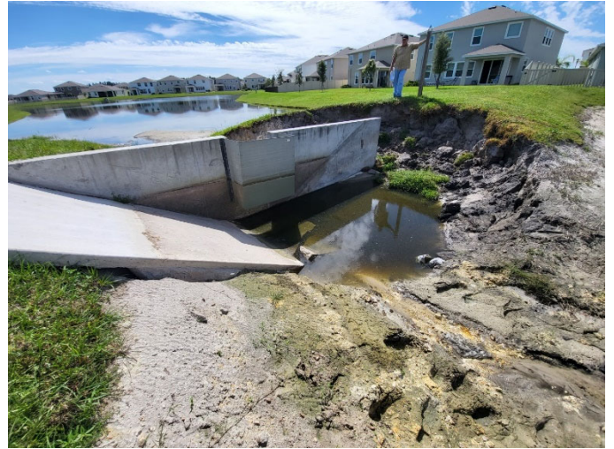
Photo showing cracks on north side of concrete structure just below the weir.
